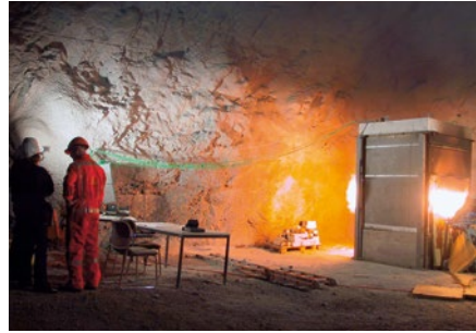
Fig. 8.5.1: In special furnace chambers fire trajectories can be replicated, panels tested and subsequently evaluated. Temperature development is measured and recorded at various depths.
