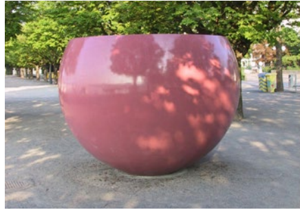
Fig. 8.12.1: Due to the development of SCC (self-compacting concrete), design and construction potential is now almost unlimited, and with special formwork technology and/or specific concrete admixtures, high quality finishes can be achieved even in the most difficult areas.
