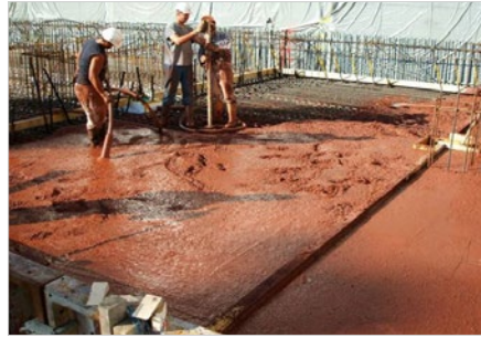
Fig. 8.16.1: The floor, walls and ceiling of this medical building were constructed with heavyweight concrete using hematite metallic aggregates to ensure full and secure radiation protection.
