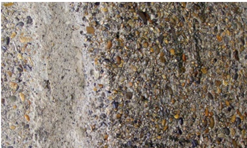
Fig. 8.7.4: Due to continuous exposure, the cement film is eroded in an initial step, and thereafter the aggregates can be rubbed, knocked or washed out of the hardened cement paste.
