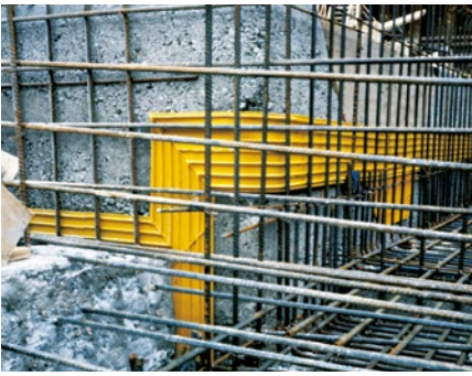
Fig. 8.1.2: Sika waterbars are flexible preformed PVC waterstops for the waterproofing of both movement and construction joints which can be subjected to low and high water pressure.
