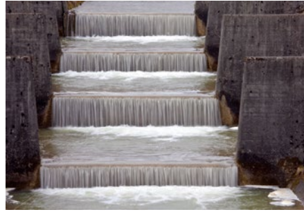
Fig. 8.71: Particularly in whitewater, concrete surfaces are subject to massive additional strains by rubble, sharp edges and abrasion, as well as possible temperature stresses due to frost exposure.
