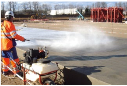
Fig. 8.10.2: Immediate coverage or curing of concrete surfaces exposed to the elements is the most crucial step for protection of such surfaces.
