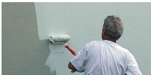
Fig. 8.8.2: As resistance of concrete against chemical attack is limited, protective coatings are often used for external protection. Epoxy resin-based protective coatings are applied over the entire surface following reprofiling of the concrete surface with sulfate-resistant repair mortar enhanced with synthetic material.
