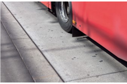
Fig. 8.7.2: Concrete roadways and other publicly accessible areas, especially those experiencing high volumes of traffic or concentrated loads, are subject to high mechanical loads and strong abrasion, often resulting in the risk of a smooth, slick surface.
