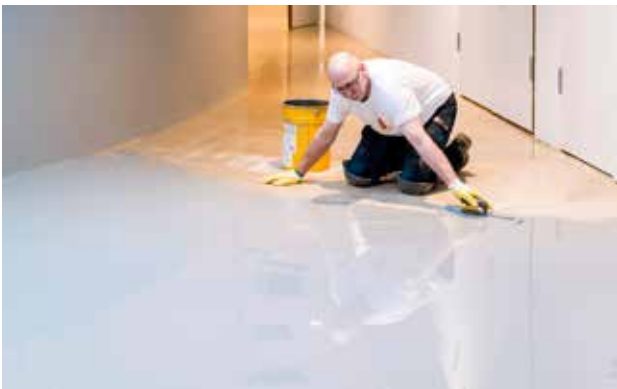
STEP 3. Self-leveling materials are applied in one or several layers to create a seamless base. Experts will pour and distribute the liquid material by using special squeegees, hand trowels, stand-up trowels and spike rollers in the process to assure a perfectly even and smooth surface.
