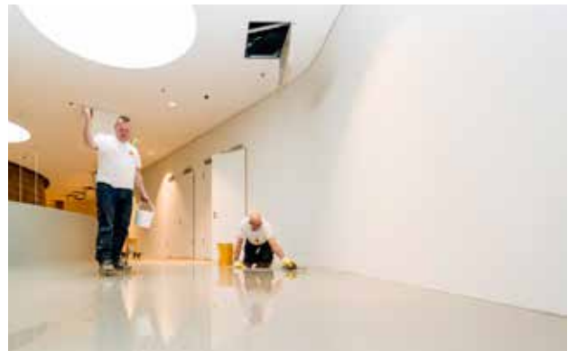
STEP 4. A wide selection of liquid resin products is available in an almost unlimited amount of colors to address many types of use. Decorative flakes or anti-slip aggregates may be broadcasted into the wet surface.
