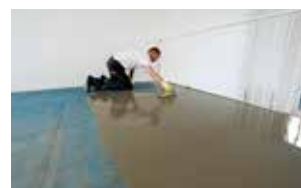
Leveling solution for perfectly even and smooth floor substrate. Page 54
