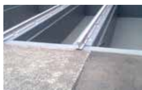
Solutions for Secondary Containment Areas. Page 40
