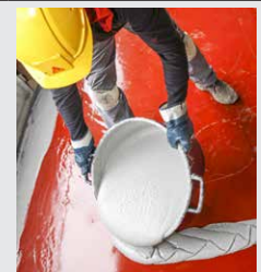
Fig. 7 Pouring the SikaTransfloor®-352 (SL/ST) to the floor
