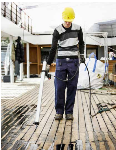
Fig. 17 Applying Sikaflex®-290 DC PRO
