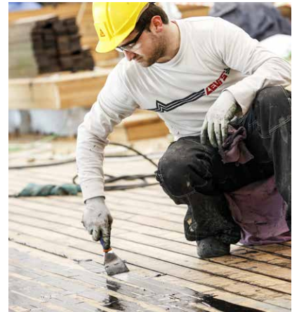
Fig. 19 Compressing Sikaflex®-290 DC PRO with a spatula
