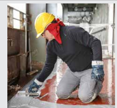
Fig. 8 Spreading the SikaTransfloor®-352 (SL/ST)
