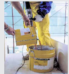
Fig. 6 Transferring the SikaTransfloor®-352 (SL/ST) to another container
