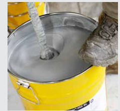
Fig. 5 Mixing SikaTransfloor®-352
