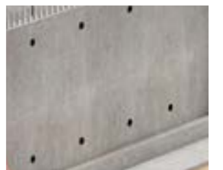
SikaSwell® Rings and Plugs Sikadur® 31 Sealing tie bar holes
