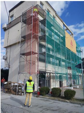
There was a requirement to refresh and decorate some parts of the façade. Sika supplied the necessary quantities of SikaColor®-650W, a waterproof, elastic and breathable 1-C paint, which is water-soluble & acrylic-based and especially designed for protection and decoration of facades.
