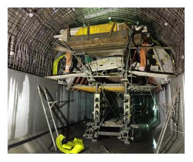
For the waterproofing of the junction point of the tunnel inlet with the metal pipe ending at the energy generating turbines station the products Sika® Injection-105-RC & Sika® Injection-201-CE.
